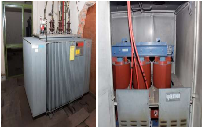
Fig. 6. a. Conventional transformer, b. Dry transformer
