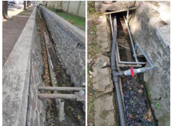
Fig. 8. Replacement of galvanic to HDPE pipelines
