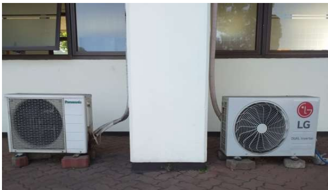
Fig. 3. a. Conventional air conditioner, b. Inverter air conditioner
