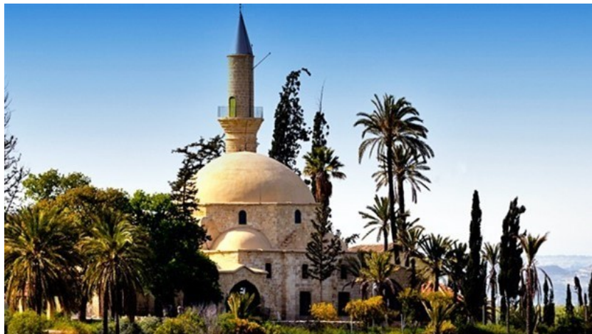
Fig. 1 Hala Sultan Mosque
