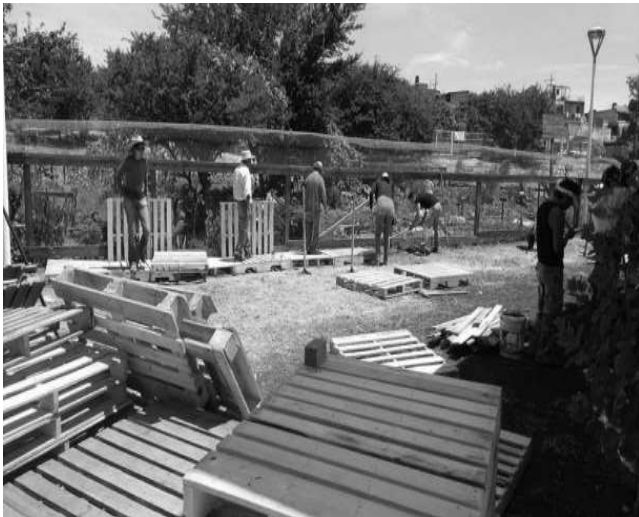
Fig. 7. PAZ construction process. Source: Traffic MAG (2016) .
